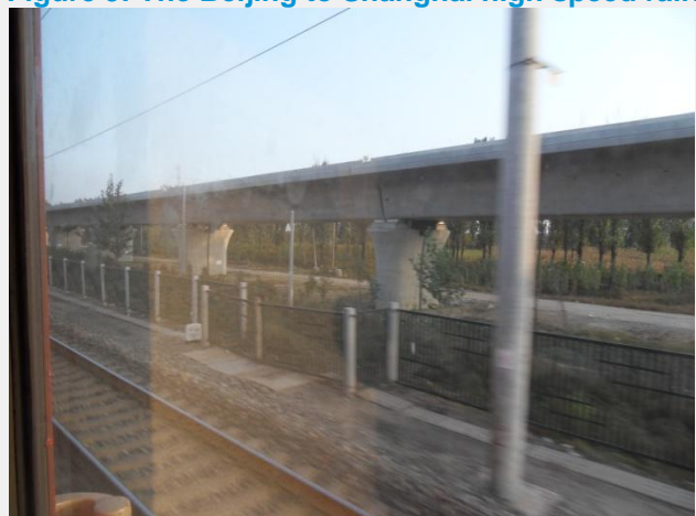
Figure 9: The Beijing to Shanghai high speed railway
