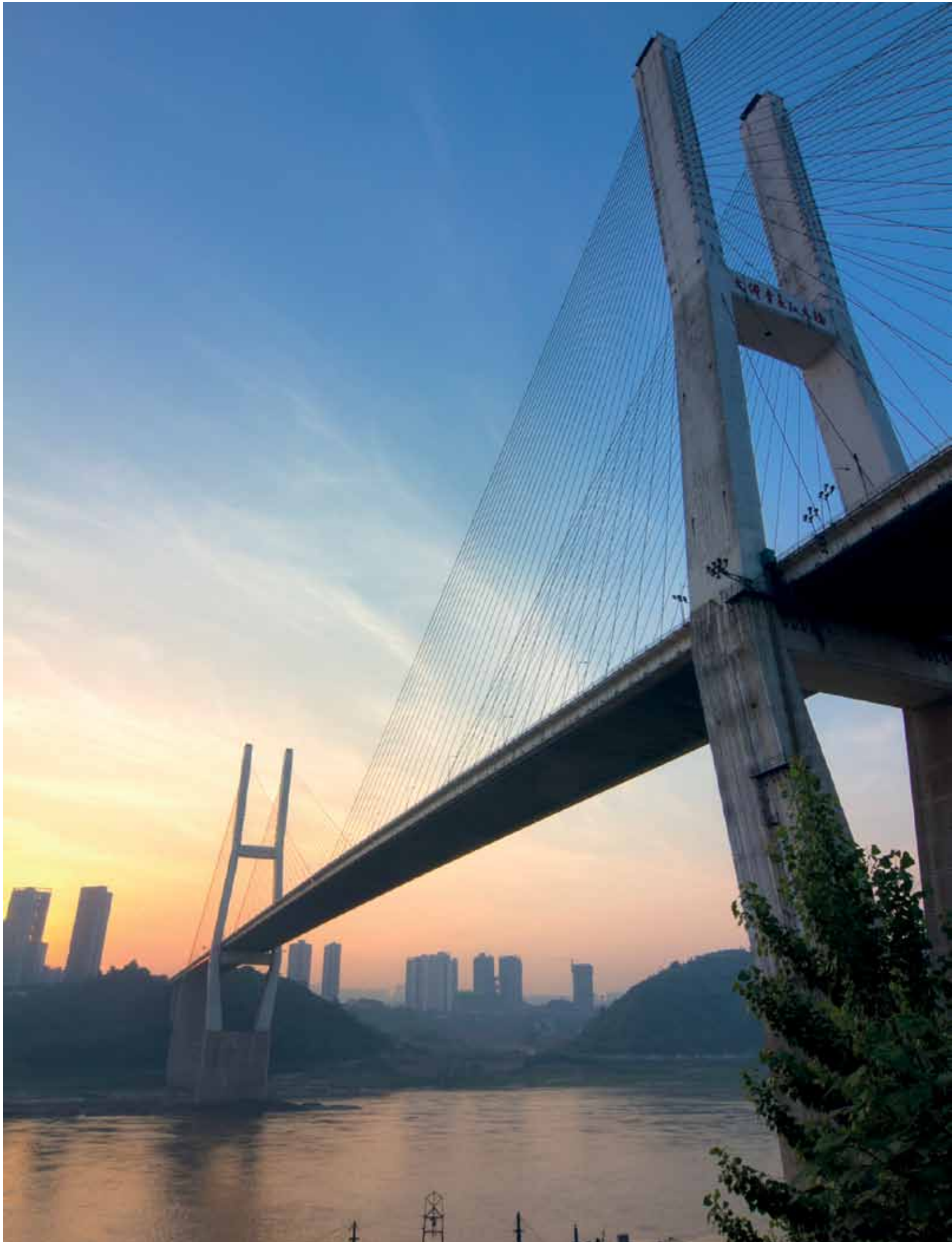
Bridge over the Yangtze River.
